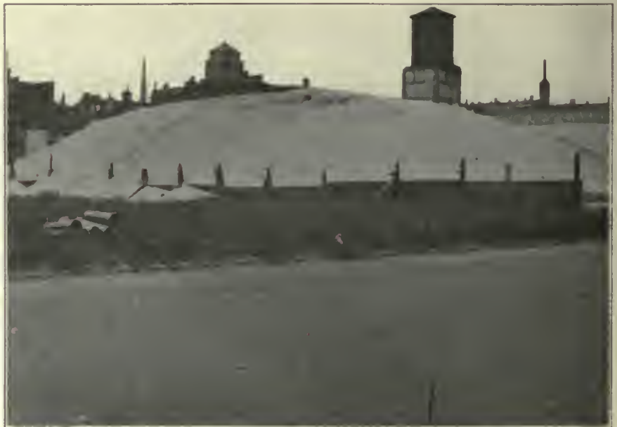
FIG. 42. EXCAVATED MATERIALS, A SOURCE OF DUST. During the construction of buildings, piles of excavated materials are frequently placed on adjoining vacant lots. The surface of such piles quickly dries out, affording the wind an opportunity to take up the resulting dust.
